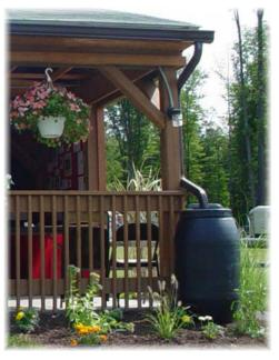
Additionally, you may also want to install a rain barrel at your downspout to capture roof runoff for use in your rain garden or other parts of your yard. The overflow from the rain barrel can be directed into your rain garden by way of a grassy swale, rock lined channel or a drip hose.
