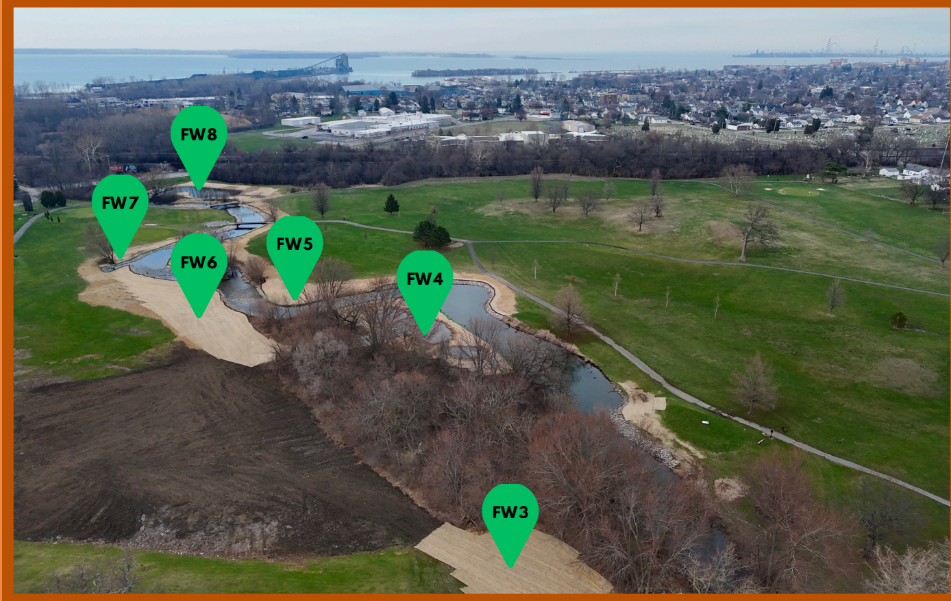
Above: designed wetlands and bank stabilization (wrapped in erosion control matting), fairway 3 regrading in progress Below: designed wetlands near Hole 5 and spoil pile
