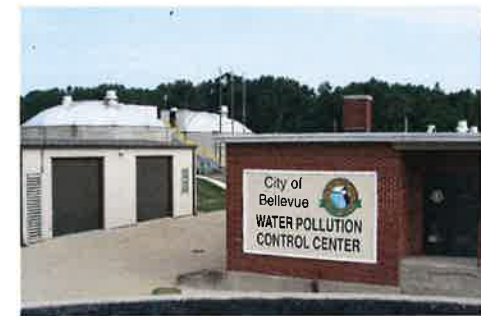
The Bellevue Water Pollution Control Center treats over a million gallons of waste per day helping reduce pollutants to Mills Creek.
